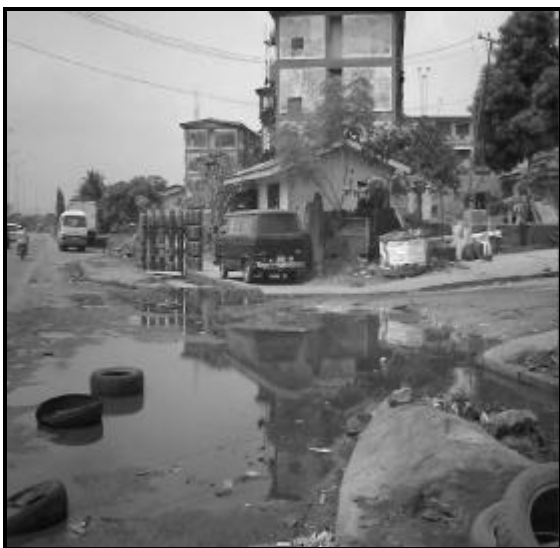
Fig. 3: Unsightly scene of a major neighborhood road water-logged and littered with used tyres.
