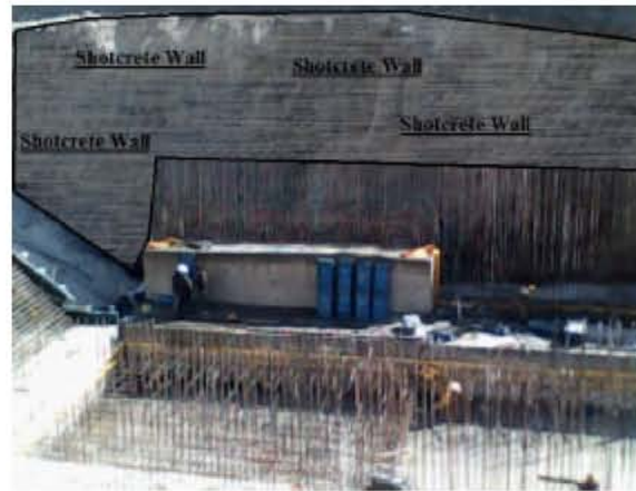
Fig. 6: Shooting concrete Wall
