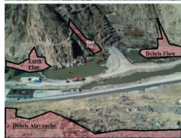
Fig. 4: Zone 4 landslide risky zones
