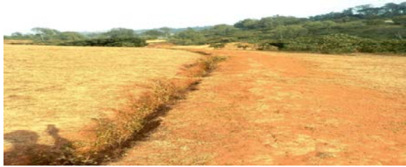
Fig. 2: Traditional cutoff drain Source [19]
