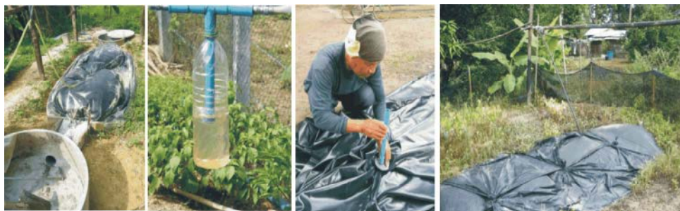
Fig. 4: The problem of the leakage of biogas and safety valve system
