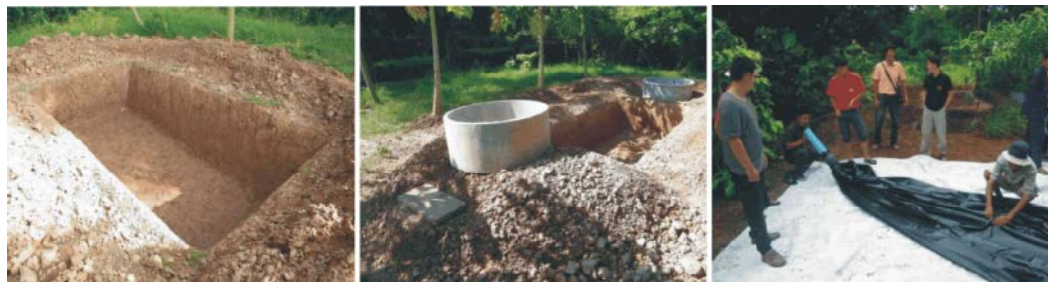
Fig. 3: The steps of balloon biogas technology constructions
