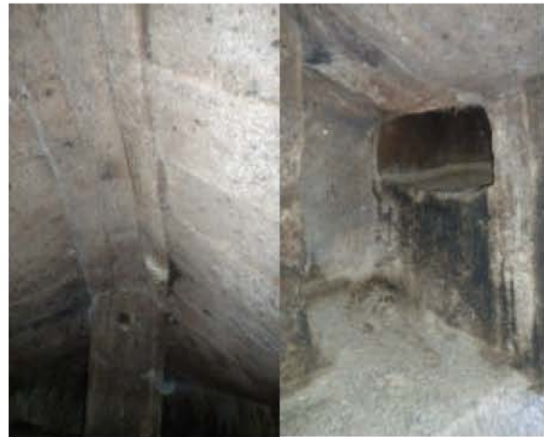
Fig. 2.17: The interior spaces of rock-carved tombs, imitating the form of a timber upper-structure, the Necropolis of Sant'Andrea Priu, Sardinia, Italia (Photo by Prof. Tancredi Carunchio, August 2010)
