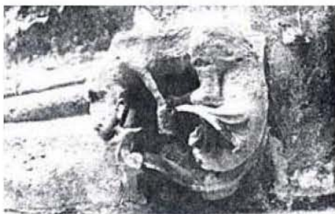
Fig. 2: Dissolution occurred in sculpture on the Lincoln Cathedral (England). Upper photo was taken in 1910. In the lower photo, was taken after 74 years, in 1984 [3]
