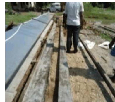
Fig. 4: Prestressing Procedure and Cast Specimens (PSC & PSGPC Poles)
