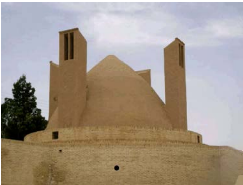
Pic. 9: Underground water reservoir in Meibod (Iran)
